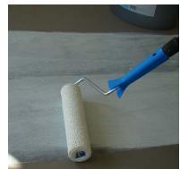
5. Apply adhesive evenly and fully to subfloor, forming a complete adhesive film. Avoid adhesive pools.
