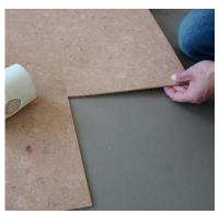
8. Lay down further cork tiles to fit and knock tightly with a rubber hammer.
