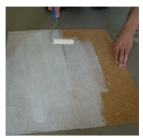
3. Apply adhesive evenly and fully to cork backing, forming a complete adhesive film. Avoid adhesive pools
