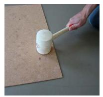
7. Lay down the cork tiles to fit and knock tightly and completely with a rubber hammer to ensure a complete bond formation.
